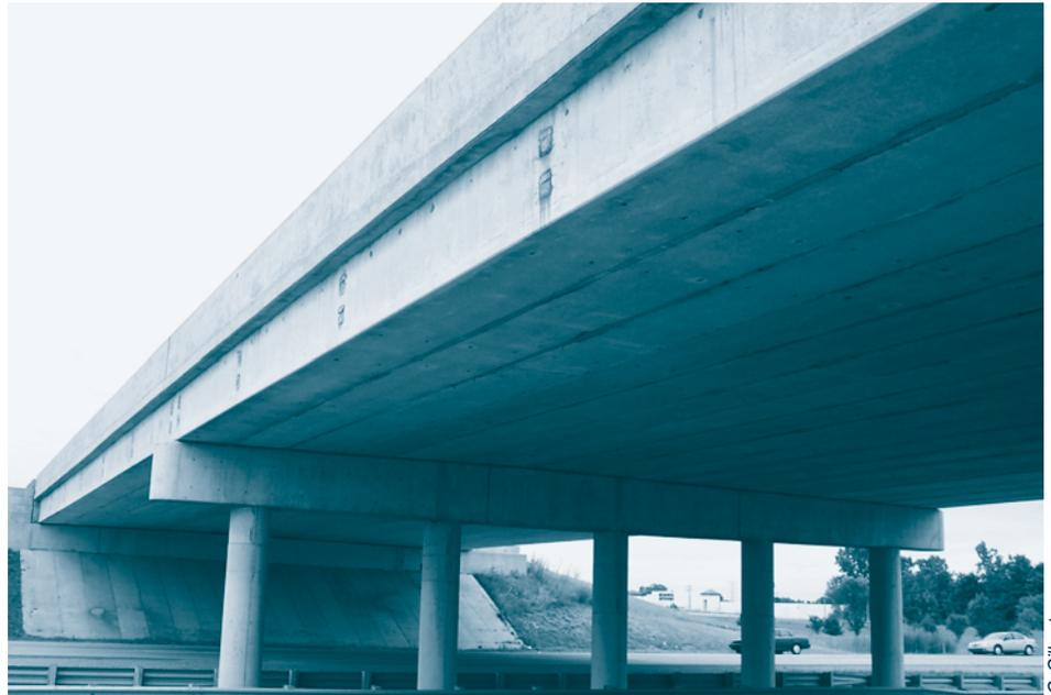
*Prestressed concrete bridges, such as the side-by-side prestressed concrete box beam bridge shown above, are among those that can be load rated with AASHTOWare's Virtis software. Other bridges (simply supported or continuous) include reinforced concrete, timber, and steel. MDOT purchased a "super-site" license for Virtis that allows local road agencies and consultants in Michigan to use it free of charge to load rate Michigan bridges.*
