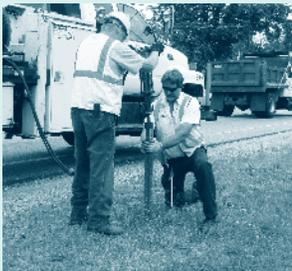
Using a truck-mounted hand-held hydraulic jack-hammer, the crew drives a 36-inch long sign base into the earth. The jackhammer eliminates the need for a boom or a bucket on the truck, and also minimizes problems with overhead obstructions. The sign base is two-inch square, heavy-gauge steel with 3/8-inch holes drilled every inch. To stop the sign post from sliding through the bottom of the base, they insert
