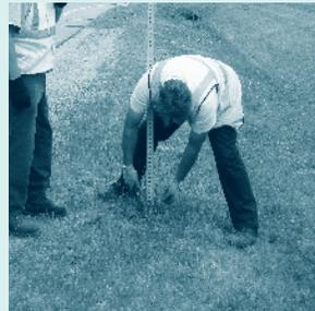
Two more sharp blows with a sledgehammer on a 3/8-inch aluminum drive rivet secures the sign post to the base.
