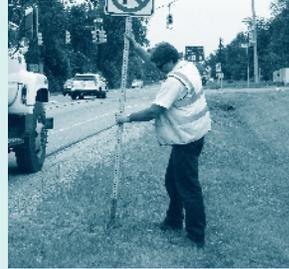
Slipping the 1 3/4-inch square, high-carbon square steel sign post into the base nearly completes the operation. The combination of high carbon steel and 3/8-inch holes every inch provides breakaway protection and meets FHWA roadside requirements. The
