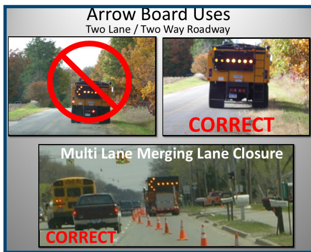
Correct uses of arrow boards on various roadways (Photo: Courtesy of Bruce Gasaway)
