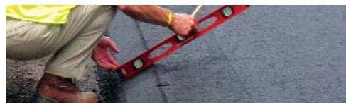
The Shoulder Wedge Maker™ (SWM) manufactured by TransTech Systems, attaches to a paving screed to create a 30-degree
