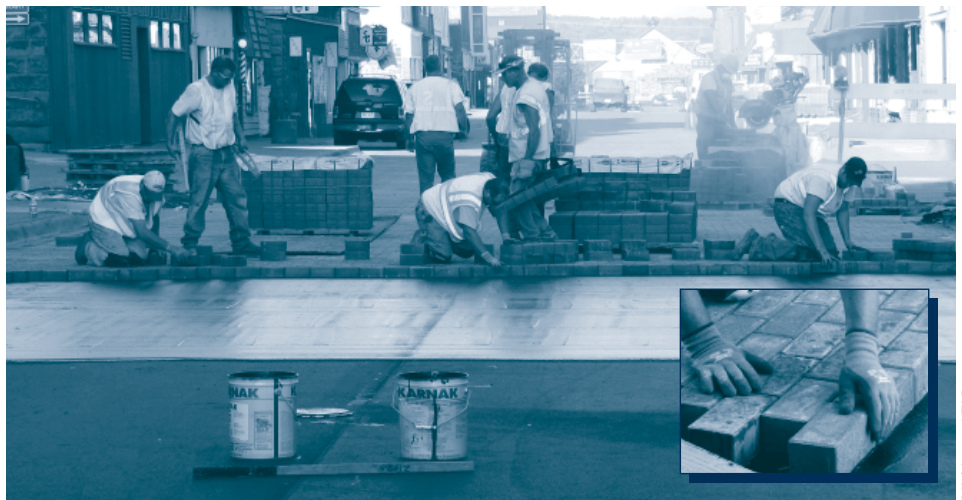
The new street surface is made up of approximately 500,000 bricks, each of which was hand-placed onto a layer of rubberized asphalt cement adhesive over four inches of asphalt pavement. The joints between the bricks were filled with a sanded grout that contained a small amount of cement to prevent water infiltration.
