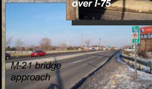
M-21 bridge over I-75
