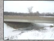
I-69 at Cox-Doty Drain
