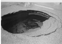
M-35 Portage Creek Bridge Cause – Beaver Dam & Flood Conditions.
