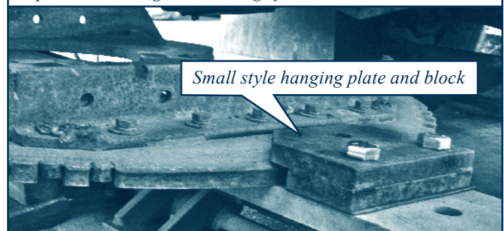
Figure 3. Turntable circle with hanging plate and block. The notches in the turntable circle accelerate wear on the hanging plate and block, causing the bolts to loosen, leading to possible binding or loosening of the circle.
