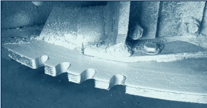
Figure 1. Turntable circle before repair. The notches seen in this picture increase wear on the hanging plate and block seen in Figure 3.
