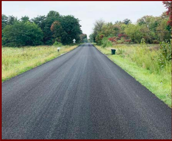
Chip sealed road in Ingham County (Photo: Courtesy of Ingham CRD)
