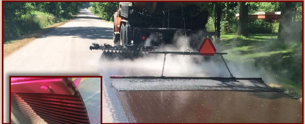
Ingham County Road Department's emulsion tail, an innovation submitted as part of the Michigan LTAP 2017 Great Ideas Challenge. Inset: Close-up view to the emulsion tail (Photos: Courtesy of Ingham CRD)
